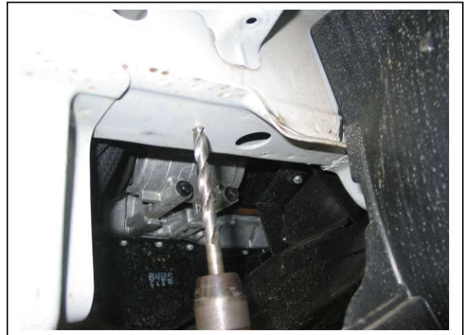
Figure 2: Enlarge holes to allow 3/8 bolts on wire for steel mount fitment.
