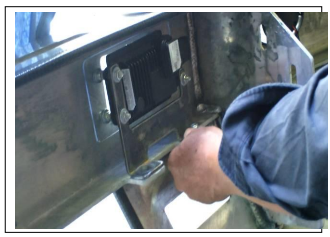
Figure 20: Attach mount to lower leg of channel
