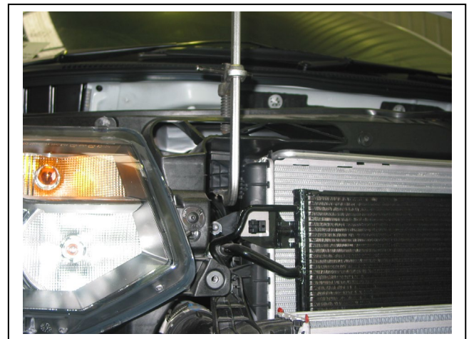
Figure 2: Supporting radiators using sliding “c” clamps under top mount. Note position of clamp
