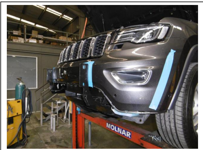
Figure 7: ECB steel mounting brackets fitted. With bumper fitted.
