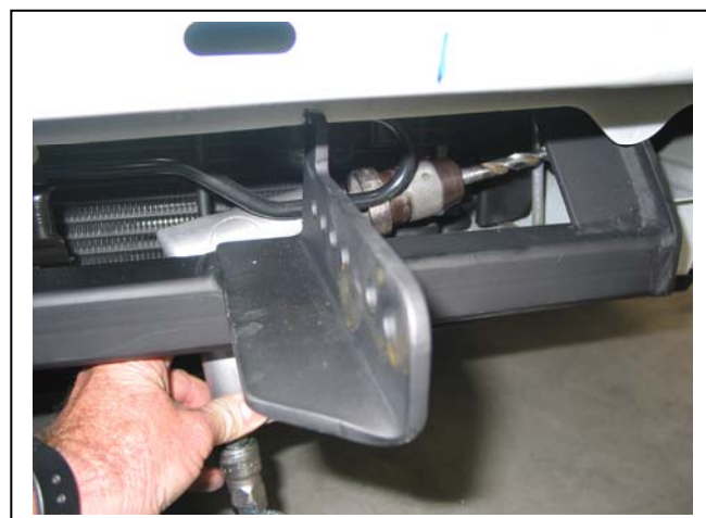
Figure 10 Showing drilling passenger side lower hole
